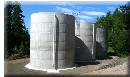
Baker Silo 30x31 reservoirs.
