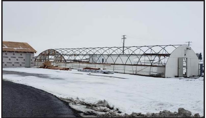
On February 1, for the second time during its life at UCA, high winds damaged the greenhouse cover. A new cover will be installed, and the greenhouse will transition to soil-based agriculture.
